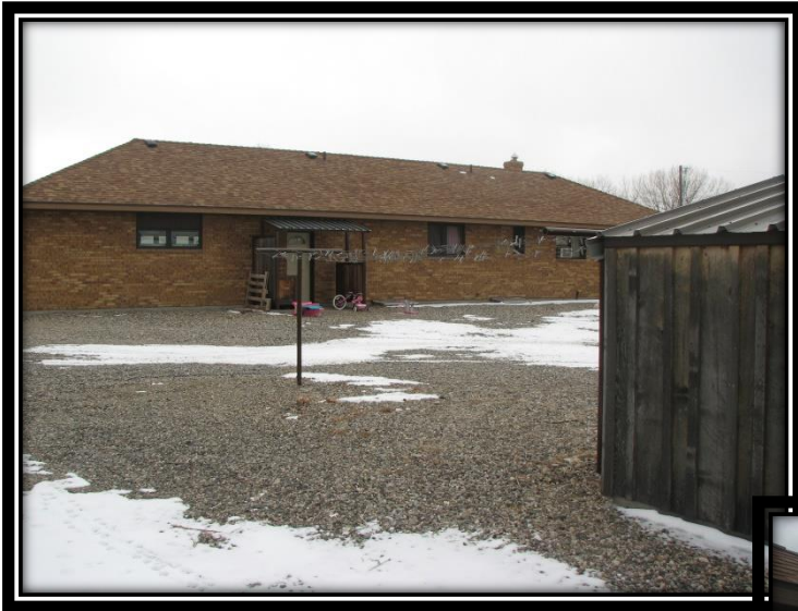
Back of Home And 3 rd Entrance
